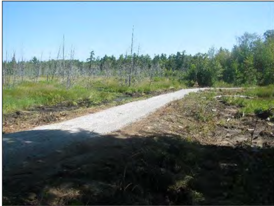
Photo 25: ATV road constructed in 2013 through the off-site wetland, facing northeast (Photo Date: August 29, 2013)
